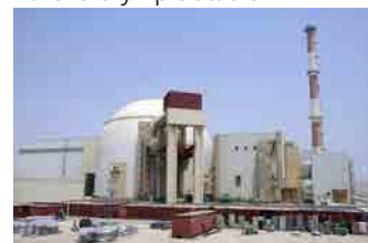
Bushehr power plant
