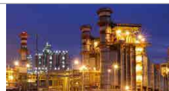
Asalouye power plant
